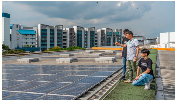
Solar panels on the rooftop of TP's buildings
