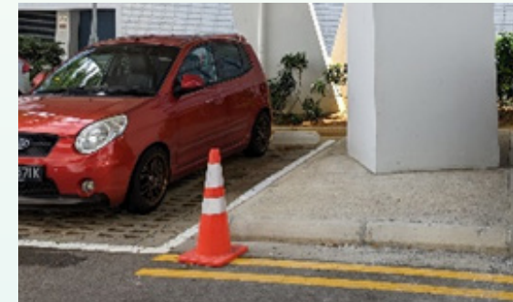
Before curb demarcation measures
