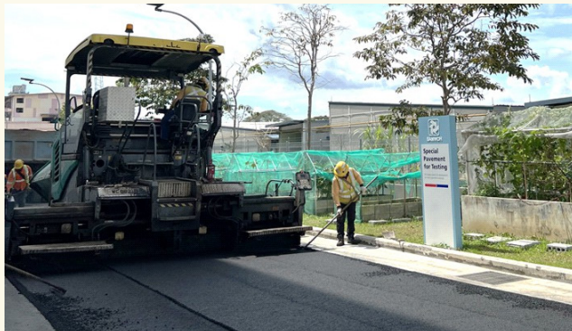
Mixed plastic modified asphalt pavement at Samwoh Smart Hub
