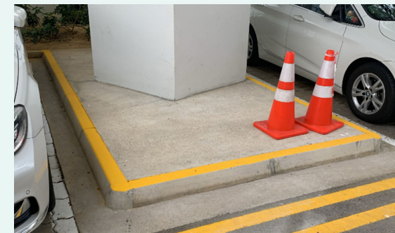
After implementing curb demarcation measures
