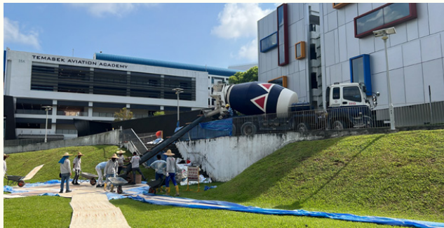
Mixed plastic aggregate concrete footpath at TP's Tembusu Garden
